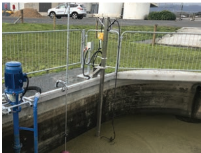
Submersible Stirrer and Lifting frame on Sump application.
