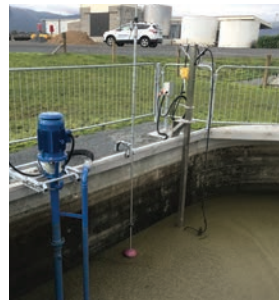
Submersible Stirrer and Lifting frame on Sump application.
