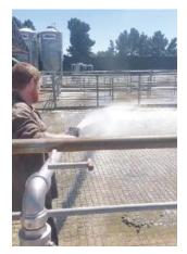
When paired with a 33l/s water pump @ 3Bar the hydrant will achieve a 20-meter radius of cover.
