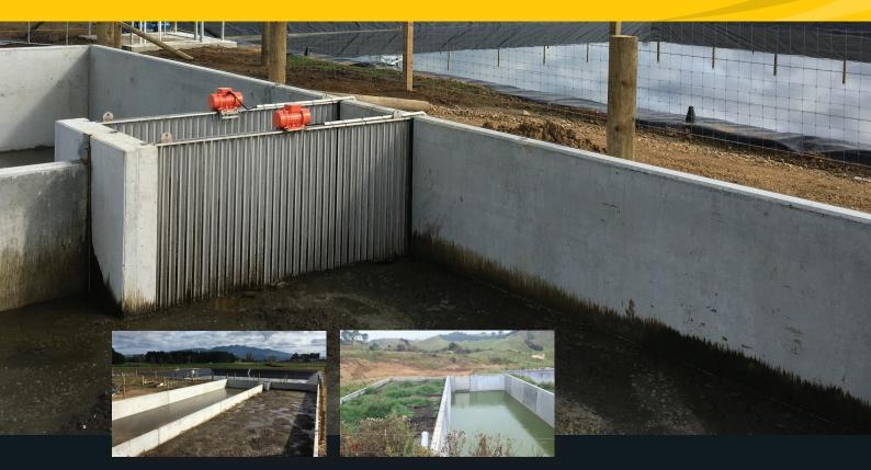
Vertical passive separation screen. Vibration clears blocked slots in screen to de-water containment.
