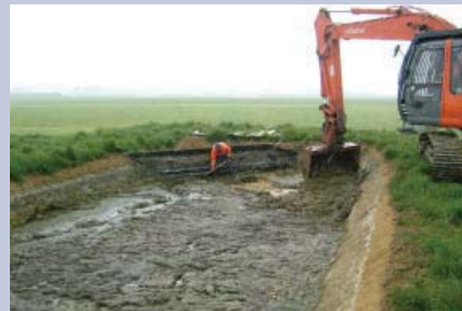
Excavator loading the dried sludge
