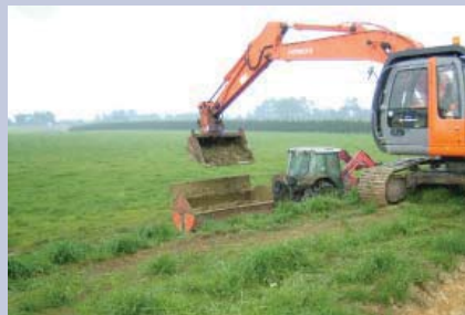
Excavator loading a muck spreader
