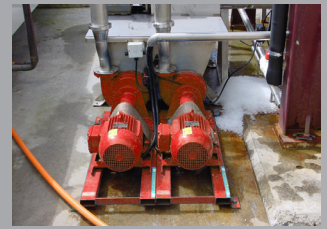
Horizontal Pumps at Chicken processing facility
