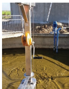
Inground Lifting Frame on Sump application.
