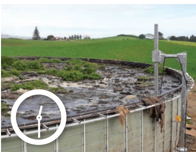
Submersible Stirrer and Over the Wall Lifting frame on Tank application. Time Lapse: 0.5hr and 3.5hr.
