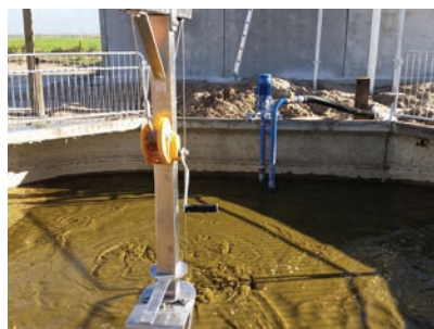
Submersible Stirrer and Lifting frame on Sump application.
